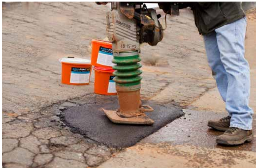
Repaired with Aquaphalt™
